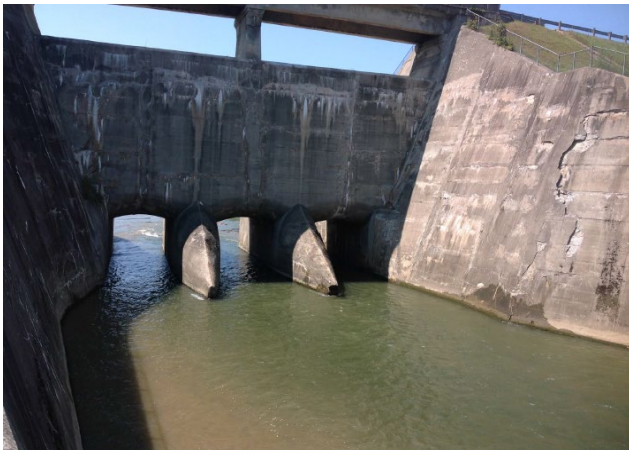
Huffman Dam conduits and spillway. Source: Miami Conservancy
